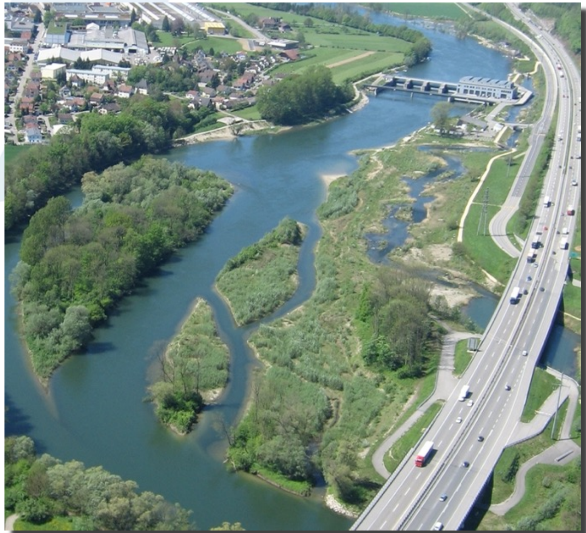
Ruppoldingen run-of-river power plant on Aar River in Switzerland
